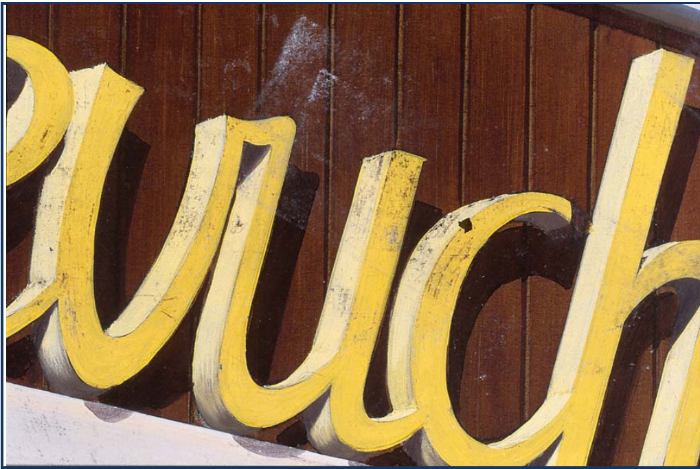
Detail - surface cleaning needed
