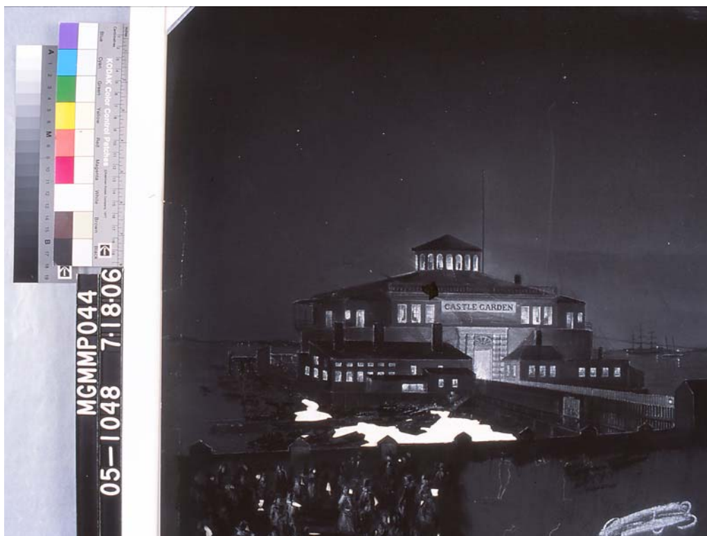
After Treatment (split repaired)
