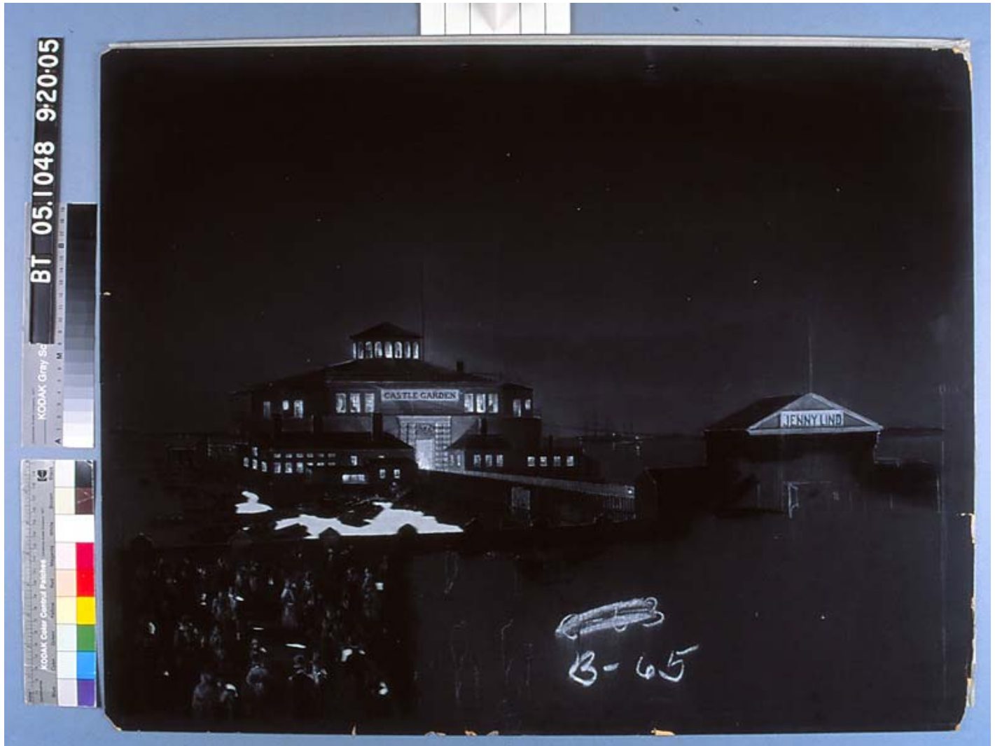
Before treatment (board is broken on left edge about half way up)
