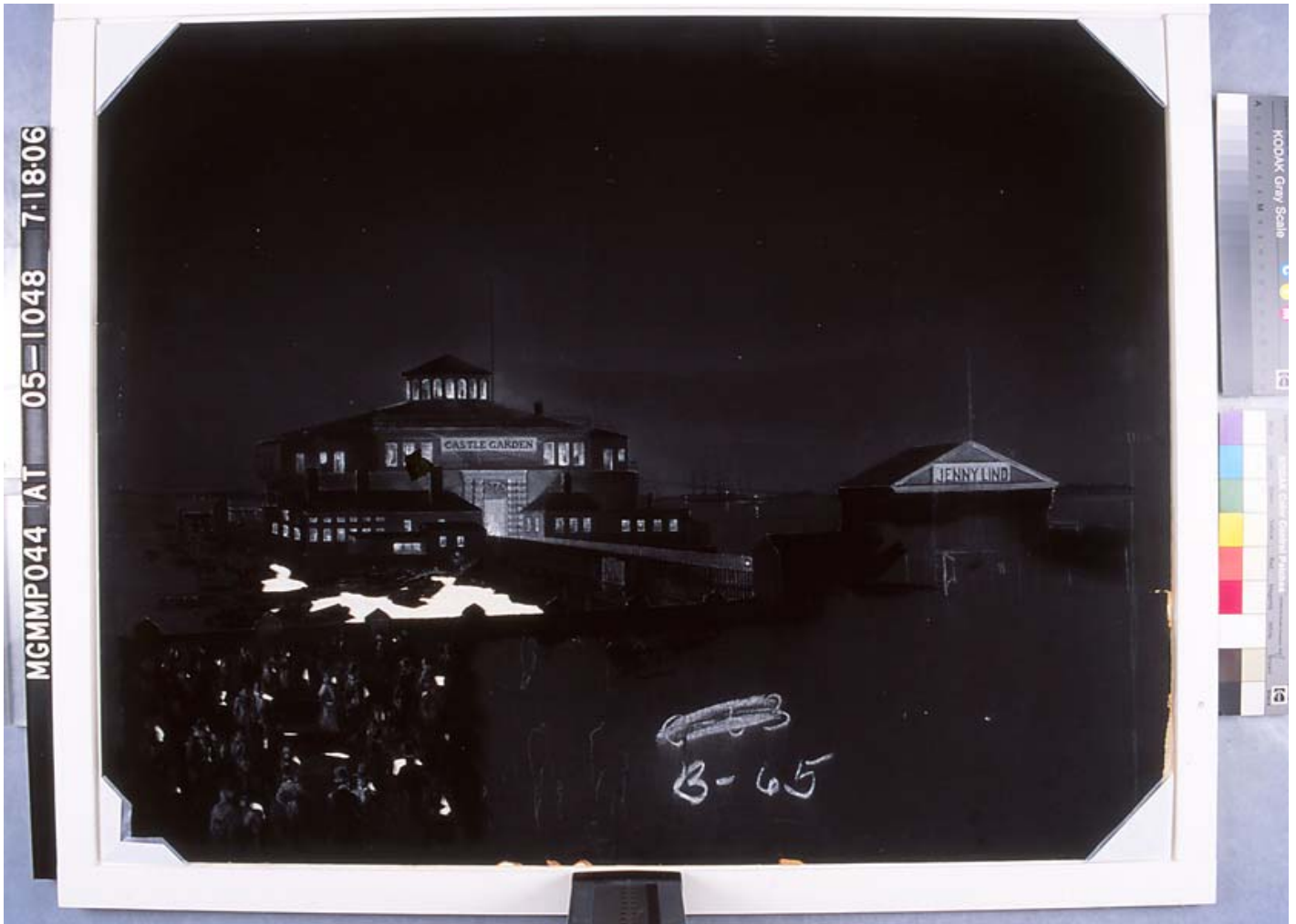
After treatment - showing board repaired
